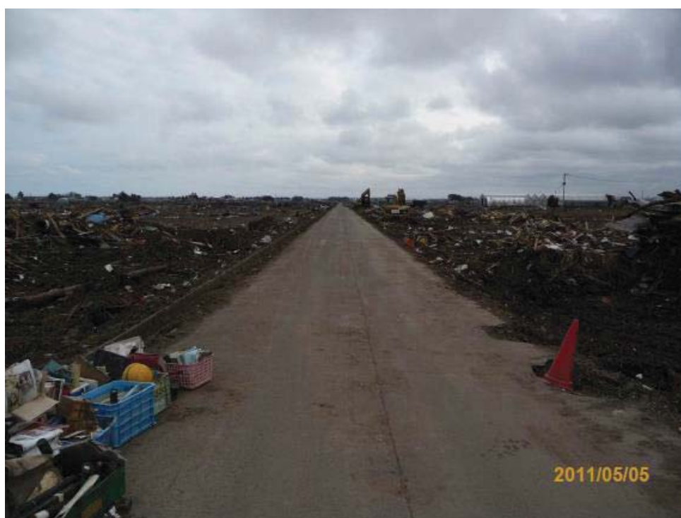
Prefectural road recovered by removing tsunami rubble in Miyagi Prefecture
