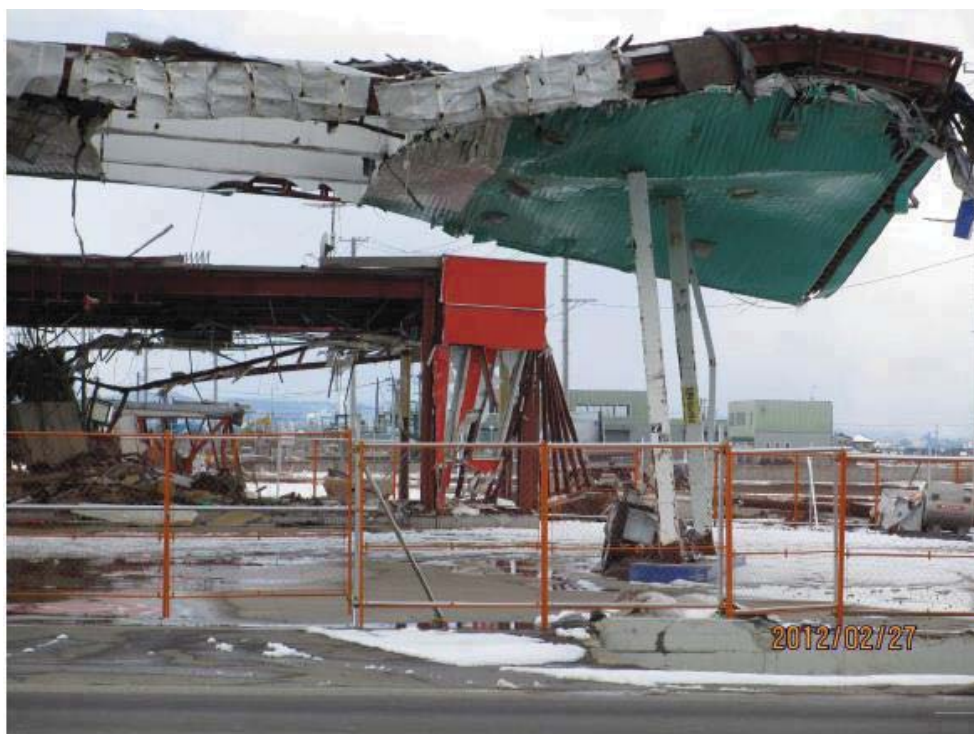
Damaged gas station by tsunami located about 1 km away from coast in Miyagi Prefecture
