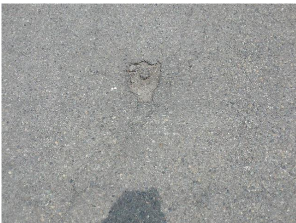
Figure 4. Example of a pothole
