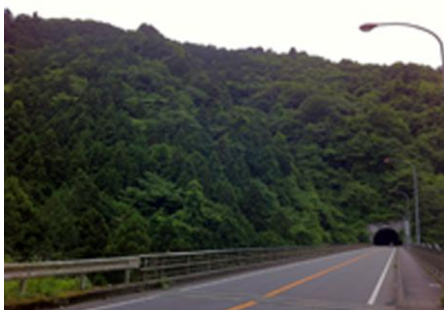
Figure26: Photograph of the right-side exit of Oosawa tunnel
