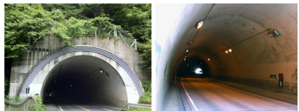
Figure19: Picture of RSSI experiment in Oosawa tunnel
