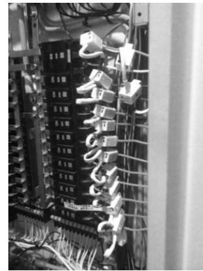
Figure 6 : CT sensors installation in power distribution panel. 14 CT sensors can be seen. The green LED shows 100v operation, LED red Indicates the system 200V operation.
