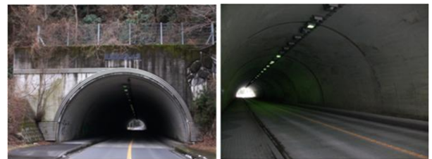
Figure18: Picture of RSSI experiment in Aikawa tunnel
